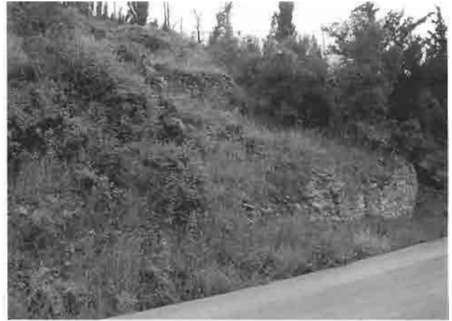
Fig. 95. The two preserved concrete pipes (in the upper left corner) leading water to the mill SM 2. The rest of the mill was destroyed when the road leading to Papatris was asphalted.
