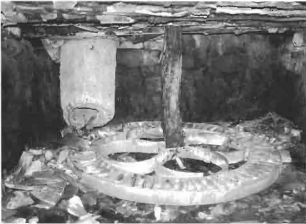
Fig. 94. Horizontal wheel of the water mill at Marmaria (SM 1). The water drops onto the spokes of the wheel through the concrete pipe, and the power is transferred back through the vertical shaft to the mill house and grinding stone above.
